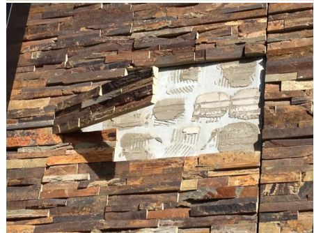
Figure 2. This cladding is a graphitic slate. As can be seen it has a dark grey and shiny surface due to Mica and Graphite (Fig 2A). The laminations are strongly bonded and the tile is quite robust and hard (Fig 2B). Provided the adhesive is not 'bond broken' by the graphite content, this cladding would be suitable for adhesive and mechanical fixing. The face of the tile is formed by cleavage plains, and the structural epoxy was applied across the cleavage/laminations.
