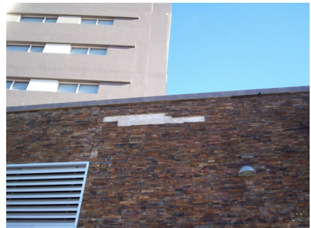
Figure 4. A final type of stacked stone which has given trouble since around 2009, is a layered mudstone which is marketed as slate. The surface is normally a brown and rusty colour as seen in Fig 4a, and side views show the fine grey laminations.
