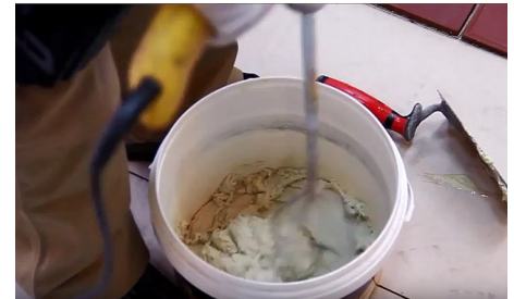
Mixing in the filler powder
