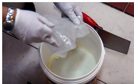
Mixing the combined Parts A+B resins and then adding the filler powder.
