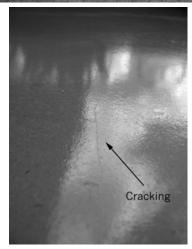
heated subfloor which has had a smoothing cement applied, and then sealed. The heating cables created a series of parallel cracks across the floor. When the floor is covered with a floor covering, these cosmetic cracks are not visible.
