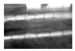
This floor shows shrinkage related cracks due to product installation problems.
