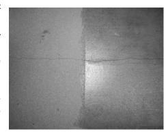
The example above shows a topping cement that has been sealed with a clear polyurethane sealer. Movement at a floor joint has produced a fine crack which is accentuated by the sealer. Cracks like this have no effect on the topping performance and are not seen when a floor covering such as carpet or vinyl is used.
