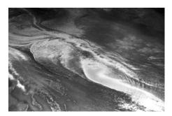
This is a sealed floor which has been subject to over-watering during smoothing cement installation. Whilst this is an attractive swirl pattern, it also highlights softer and weaker areas defined by the white patches. Also note the sanding marks made in the surface to 'finish' the floor before being sealed.
