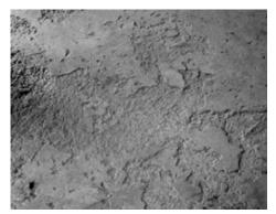
The concrete surface has a layer of laitance which needs to be removed back to the sound material underneath.
